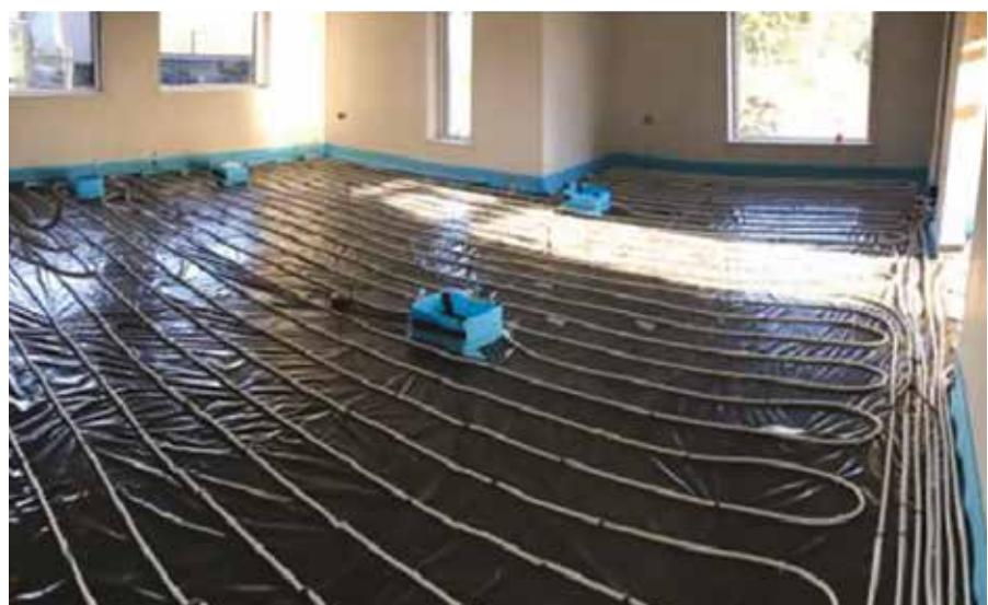
Finished preparation should be completely water tight to prevent leaking, polythene and other materials should be grease free and sitting flat to the insulation boards and all pipes and conduits running in the screed must be fully secured.
